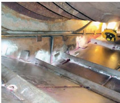
*Exhaust plenum repair materials fabricated by AAF, shipped to platform and installed in situ*
