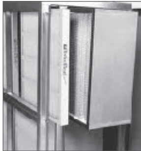
2" PerfectPleat® pleated filters are shown installed in the prefilter track on the upstream end of the housing in front of AstroCel® HCX final filters.
