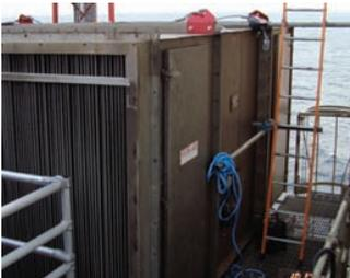
Exposed double sided air intake filtration unit on FPSO
