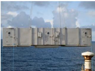
Single piece lift of double air intake unit during installation
